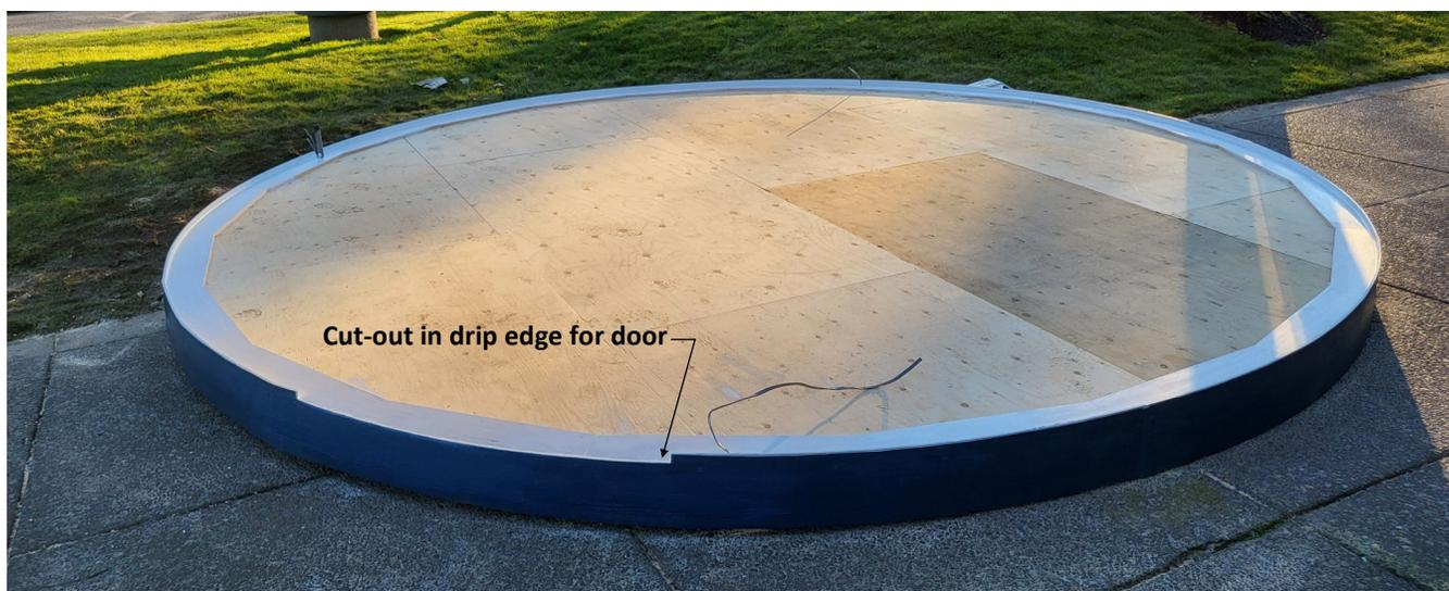
The drip edge should be inspected and maintained from year to year. If it starts to deteriorate or rot it will need to be replaced before water can infiltrate the platform's framing and cause further damage.
