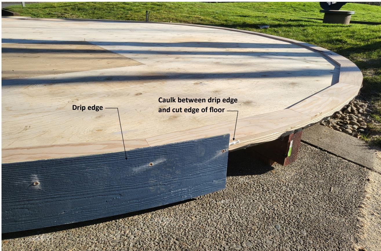
The bottom portion of the drip edge will be exposed and visible once the yurt is installed, so it should be stained or painted to protect it and to match the exterior color scheme. Metal flashing can also be used over the drip edge for further protection from the elements. Also keep in mind that the 1" portion of the drip edge that extends above floor level will be visible on the inside and can be painted or stained to match the interior color scheme.
